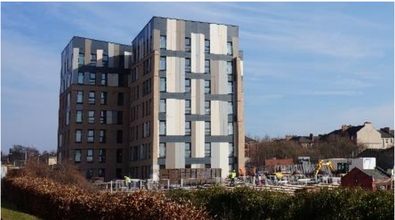
Figure 4. Construction work at Yoker.
