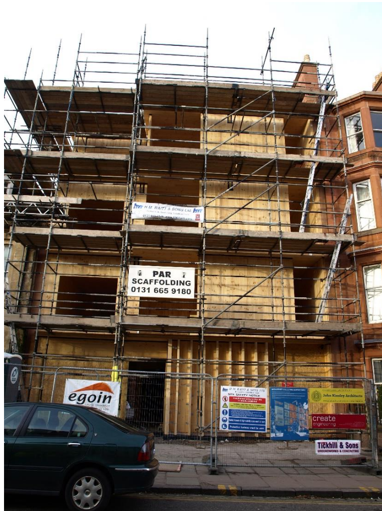
Figure 5. The Portobello project during the construction phase.
